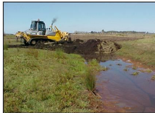
Filling in the old drain.
