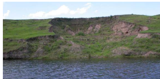
Plate 3.1 Rotational Slump Failure
