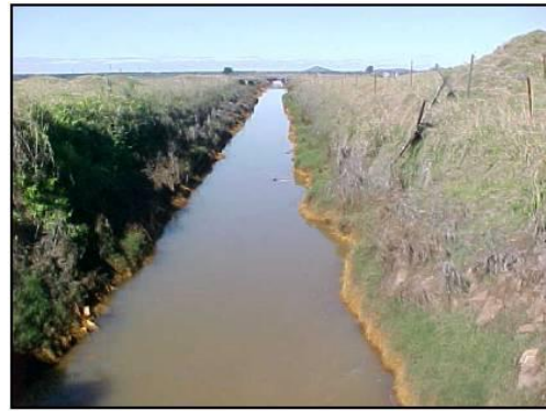
Historical deep drainage system.
