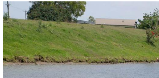
Plate 3.2 Bank Notching by Wind / Boat Waves
